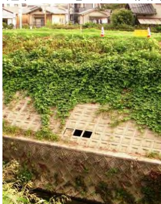
⑦小畑川支川犬川堤防 2
